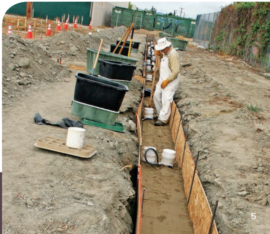
Daniels Street horizontal extensometer under construction.
